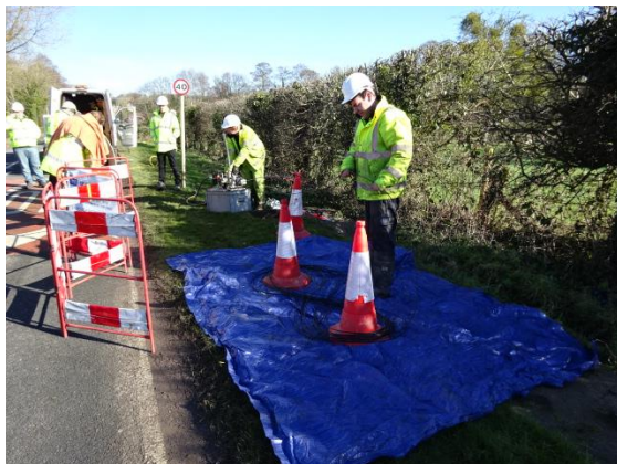
Figure 11. Cable Fleeting For Centre Blowing
