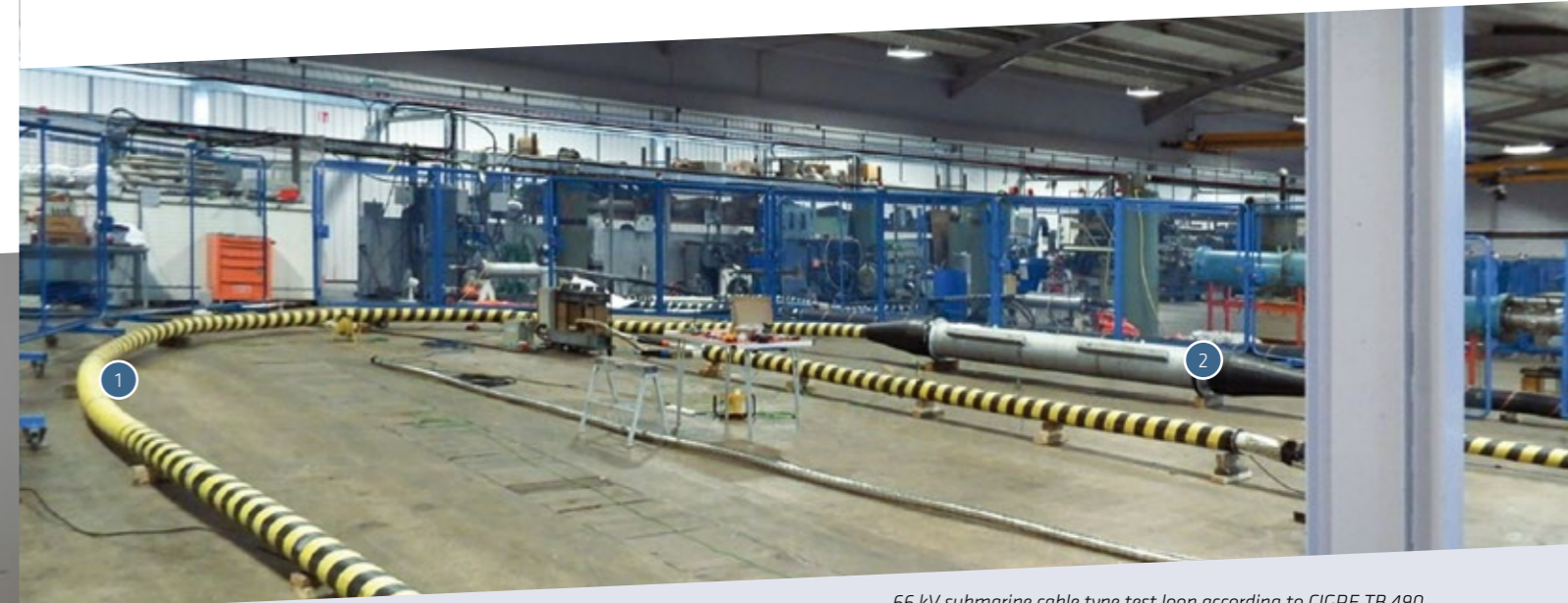
66 kV submarine cable type test loop according to CIGRE TB 490
